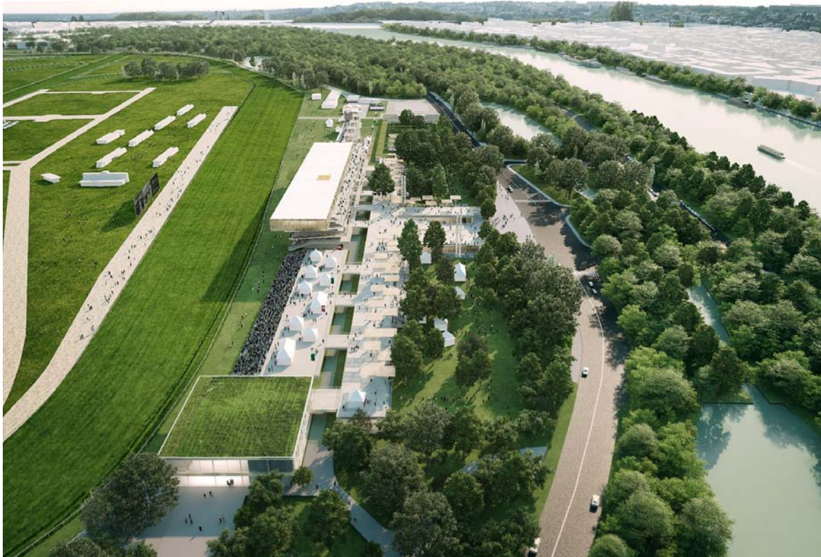
Aerial view from the Seine river
